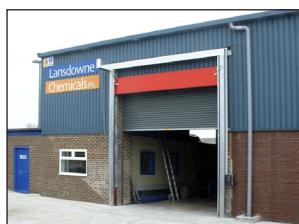
Automatic drop-down barrier.
