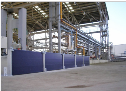
Multi-span 900mm high removable containment barrier.
